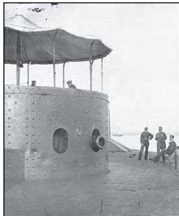
When constructed in 1862, the *Monitor's* rotating gun turret was the first of its kind. While John Ericsson, *Monitor's* designer, was not the first to envision a revolving turret, his design was the first completed. The turret is 21.5 feet in diameter and nine feet tall. It was constructed of eight one-inch thick iron plates and weighed about 120 tons.
