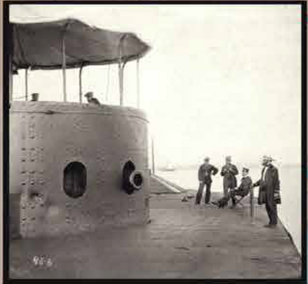
Several of Monitor's officers standing on deck; dents on the rotating turret from the March 9 battle clearly visible.
